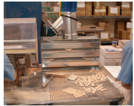
A stationary dust collection hood at a fill station in the filling room pulls in fugitive dust created during the container-filling process.
