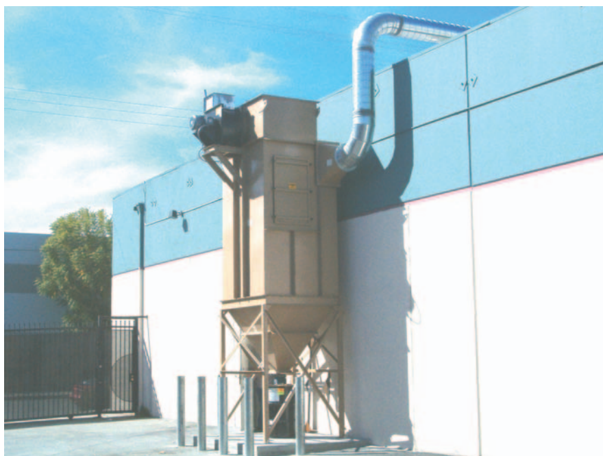
The baghouse dust collector, which uses 40 fluorocarbon-treated oleophobic bag filters for a total of 378 square feet of filter media, operates with an air-to-cloth ratio of 9.8-to-1.
